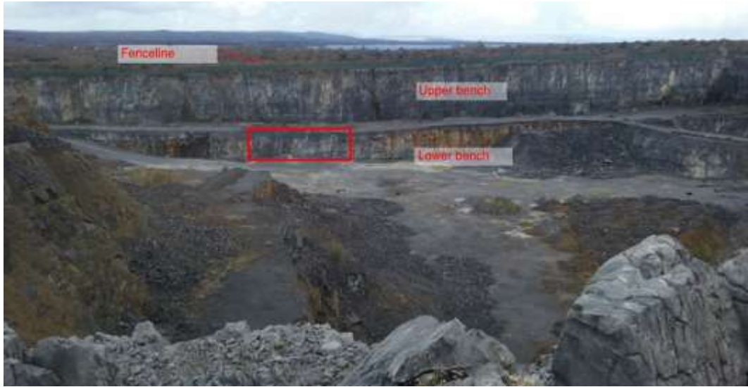
Figure 3.4: Features of the eastern tunnel portal area, with extent of tunnel portal marked within red rectangle
