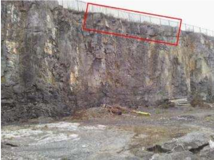
Figure 5.2: Wedge failure in the upper bench
