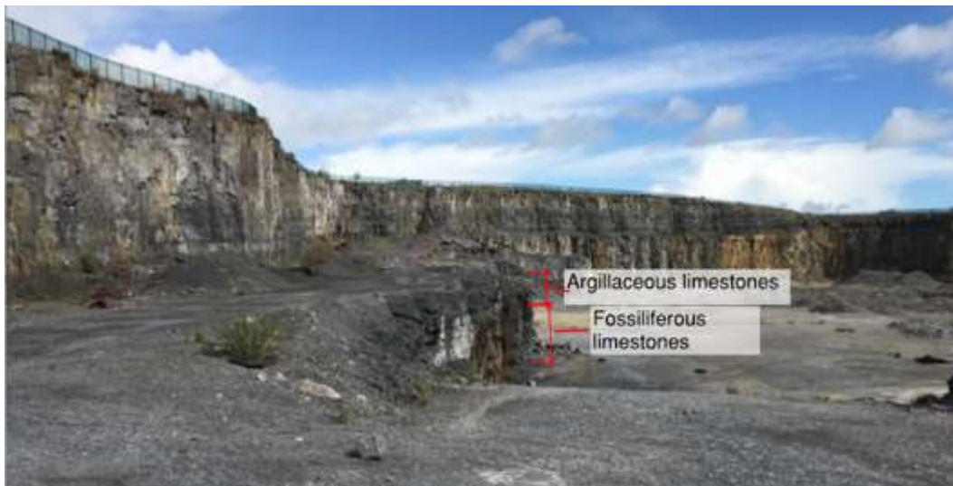
Figure 3.14: Cyclical sequence of Limestones at Lackagh Quarry
