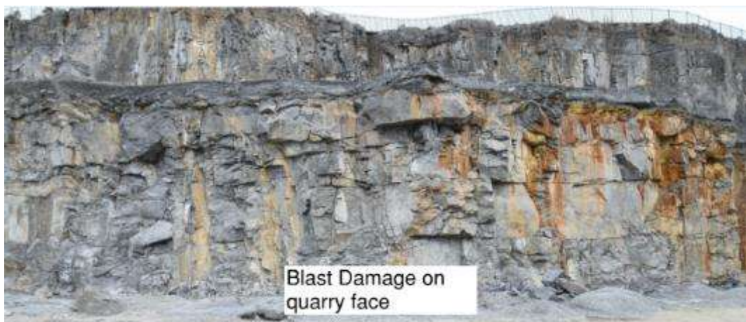
Figure 3.17: Blast damage on quarry face
